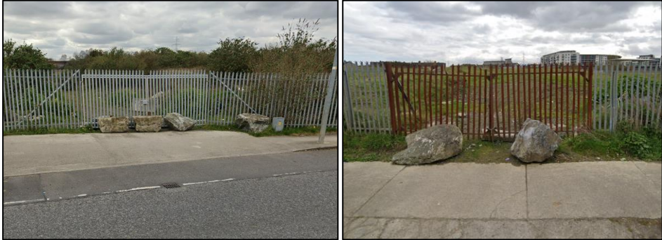
Figure 5 | Site 4 (left) & Site 5 (right) Existing Access Points
